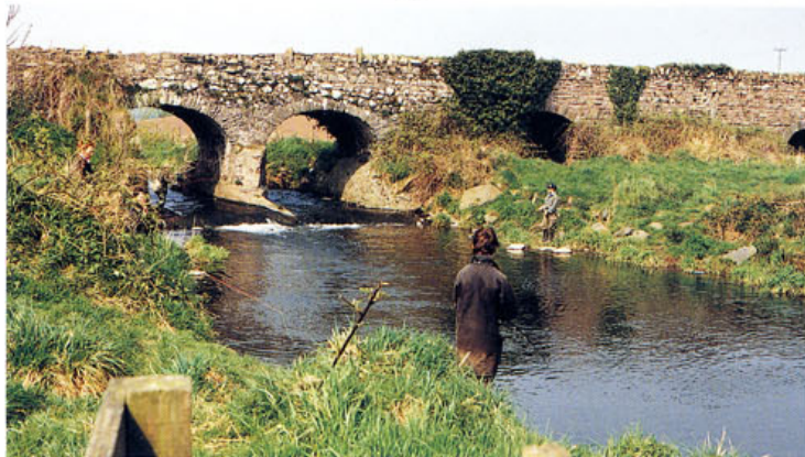
Hoping for a bite at the old five-arch Kennel Bridge, demolished in 1995.
